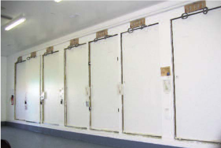
FIG 7 Interior of NET Facility
