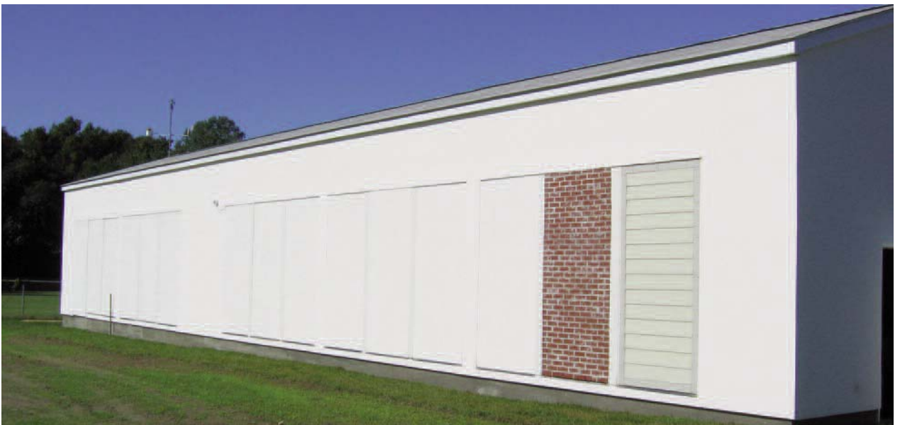
FIG 8 Exterior of Southeast Wall NET Facility (Phase 1)
