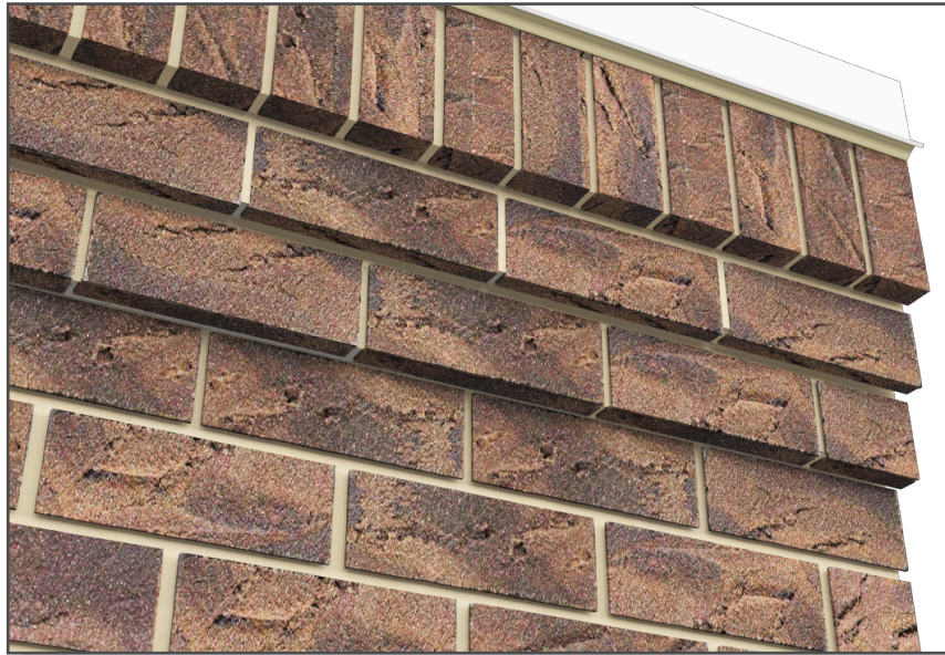
Inset 1 Bottom Side of Cornice
