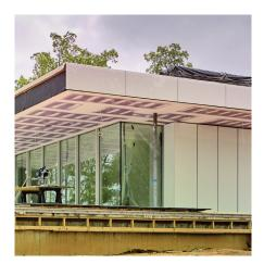
Part of the Ventec<sup>™</sup> manufacturing process includes the fusion of color onto the back of the glass. The hues melt into the glass, creating permanently colored panels that will not wear, scratch, fade, or incur water damage. Vivid colors and different panel sizes are available as options, offering many aesthetic choices for either new-build or renovation.
