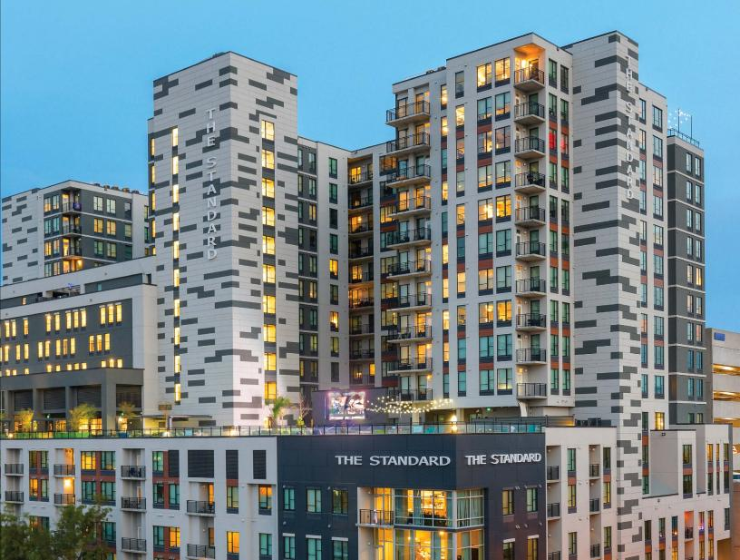
StoPanel and Pella Windows have teamed up to develop a new concept - a fully integrated and tested prefabricated panel and window system. This simplifies prefabrication of complete wall assemblies by pre-installing Pella's receptor system in the factory. Fastened in the "dry zone," featuring double line sealant, and fully tested to ASTM standards to verify performance, opportunity for on-site construction defects is minimized.
