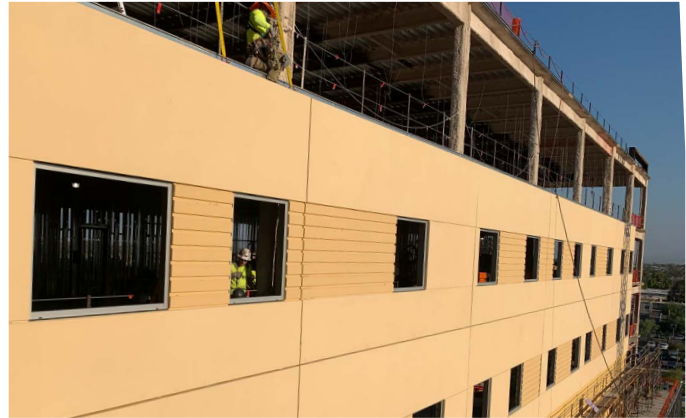
Window receptors and sealants are pre-installed in a controlled factory setting prior to delivering the panels to the jobsite.
