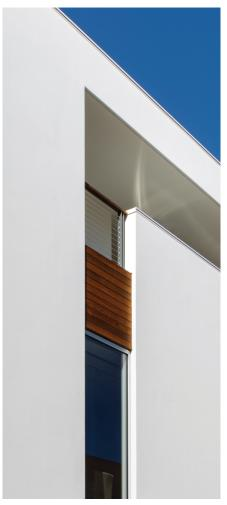
From a construction point of view. the main challenge of the project was the time needed to QA/QC the substrate to ensure it was completely flat in order not to project any bumps, seams, and/or blemishes, according to Stone.
