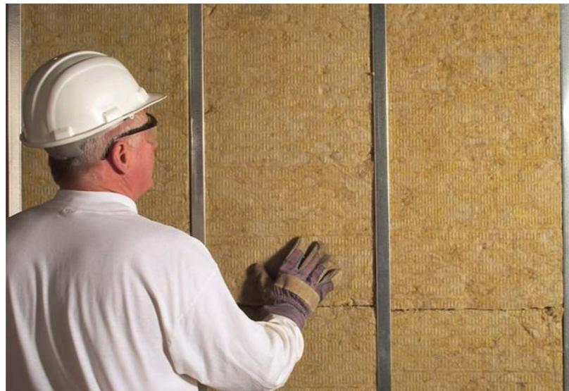
Thermafiber® Mineral Wool Insulation products are made for easy handling and installation. As a semi-rigid product that is easy to cut and install, its flexibility allows it to conform to building shapes and construction irregularities. It comes in standard-sized sheets and is easily cut with a serrated knife.
