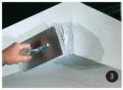
Reinforce the underside of the return area with Sto Mesh. The mesh should overlap by at least 4 in (10 cm) at the connection with the reinforced façade.
