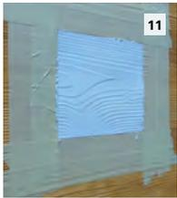
11 Insert new StoCast Wood piece into the repair area firmly pushing from side to side for full bedding in the adhesive. Adhesive should squeeze out of the joints. This will help with sealing the repair.
