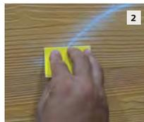
2 Using sand paper or steel wool, sand the repair area so that it matches closely to the wood graining next to it.
