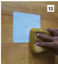
12 Remove masking tape and wipe off excess adhesive with a damp sponge. Be careful not to remove adhesive out of joint. Allow to dry.
