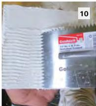
10 Apply a coat of StoCast Wood Adhesive to the back of the replacement piece, then notch using a 1/4" x 1/4" V-notched trowel.
