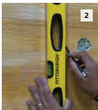
Mark the section to be removed. Make sure this is at least 2-1/2 inches (64mm) each side of the puncture in the section of this StoCast Wood plank that is being replaced.
