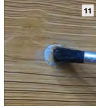
With small paint brush, apply StoCast Wood Stain to repair.
