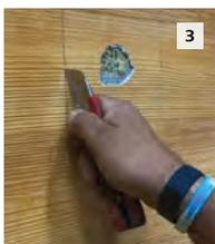
With a sharp knife, cut through StoCast Wood being careful not to cut through base coat below.
