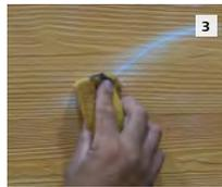
3 Wipe sanded area with damp sponge to remove any dust from sanding process. Allow to dry.
