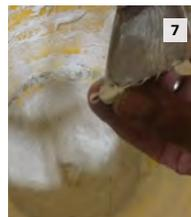
7 Apply StoCast Wood Adhesive to the back of the repair piece.
