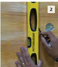
Mark the section to be removed. Make sure this is at least 2-1/2 inches (64mm) each side of the puncture in the section of this StoCast Wood plank that is being replaced.
