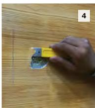
With a stiff scraper, carefully remove area of StoCast Wood. **Note: Inspect and repair any damage to underlying substrate at this time if needed.**
