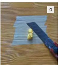
4 After TurboStick® foam is dry, shave off excess foam flush with StoCast Wood.
