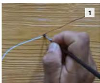
1 Clean to remove surface dirt. Use paint brush to apply StoColor Wood Stain into the scratch or defect
