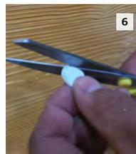
6 Using scissors, cut a circular piece of StoCast Wood around a knot texture. It may be necessary to sand the edges to ensure a tight fit.
