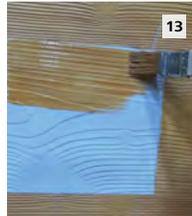
13 Using a brush, apply StoColor Wood Stain to replaced piece as per installation instructions.
