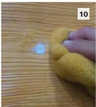
With damp sponge, lightly wipe off any excess adhesive being careful not to remove adhesive from joint. Allow to dry.
