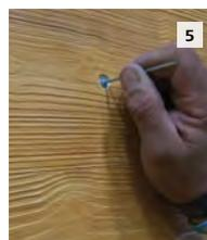
5 With the head of a nail, push in the TurboStick® foam just below the surface of the StoCast Wood. This will allow room for adhesive and patch material.
