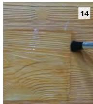
14 Blend the stain from the new to existing section. It may take multiple coats to get to the desired shade. Allow each coat to dry before the application of additional coats.
