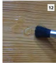
Lightly blend new stain into the existing surface. It may take multiple coats to get to the desired shade. Allow each coat to dry before the application of additional coats.
