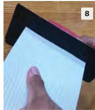
Measure and cut a piece of StoCast Wood to fit the cut-out area. It may be necessary to sand the edges to ensure a tight fit.
