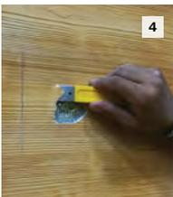
With a stiff scraper, carefully remove area of StoCast Wood. **Note: Inspect and repair any damage to underlying substrate at this time if needed.**
