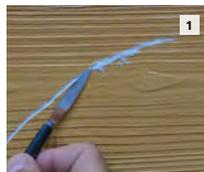
1 Clean area to remove surface dirt. Using a detail tool and your finger, fill gouged area with StoCast Wood Adhesive. Build flush or just above existing surface. **Note: this may take multiple coats.** Allow to dry.
