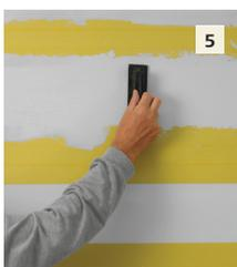
**5** Place the grain texture tool on the wet Stolit Milano and push or pull it along in a slow rocking motion.
