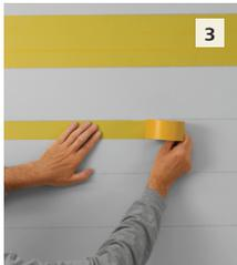
**3** Place marks at desired board widths, snap or draw lines. Mask one half of the board fields. Pay close attention to level and straightness to achieve a consistent final appearance.
