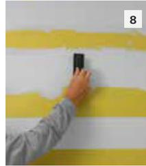
**8** Work on the remaining areas, remove the tape. Leave the surface to dry.
