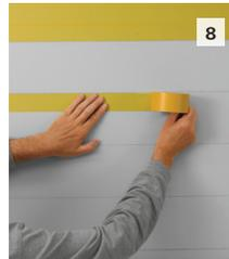
**8** Lightly sand the textured surface to remove high points to aid in the taping process. Clean the surface to remove dust, then mask already textured surface. Work on the remaining areas. Remove tape. Leave the surface to dry.
