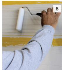
**6** Optional: leave Stolit Milano until it is dry to the touch. Level the rough edges using a dry foam roller. Applying only light pressure, guide the foam roller along the board lengths.
