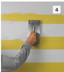
**4** Using a stainless steel trowel, apply a thin layer of Stolit Milano to one board field.
