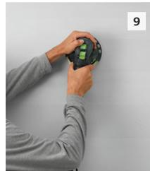
**9** Lightly sand the entire surface with a manual or power sander with a dry abrasive paper of P80-P100 grit.
