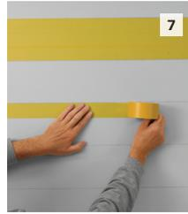
**7** Lightly sand the textured surface to remove high points to aid in the taping process. Clean the surface to remove dust, then mask already textured surface.
