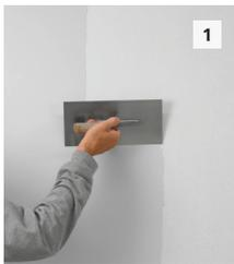
**1** Apply a smooth coat of Stolit Milano, over entire properly primed wall. Leave the surface to dry.
