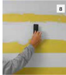
**8** Work on the remaining areas, remove the tape. Leave the surface to dry.
