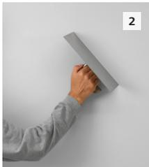
**2** Knock tips and ridges off the dried finish using the edge of the stainless steel trowel or lightly sand with a dry abrasive paper of P80-P100 grit. Blow/brush all loose particles/dust from surface.
