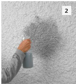
**2** One application technique is to evenly apply StoTique in patches using a spray bottle. Apply StoTique using a brush, roller or sponge. Take care not to apply them in a straight line, particularly in areas such as scaffolding platforms.
