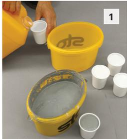
**1** Dilute StoTique with water up to the maximum amount as indicated in the Product Bulletin. Stir StoTique frequently during its application. Note: if less water is used, StoTique will be thicker. This may be preferred and more suitable to created desired effect.
