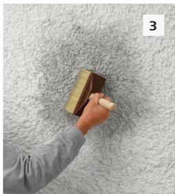
**3** Immediately smooth StoTique using a brush, sponge or a cloth. Leave the spots from the first application cycle to dry thoroughly before starting the second application.
