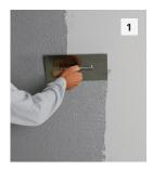
Using a stainless steel trowel, apply Stolit 1.0 and trowel off to aggregate size. Only apply finish to the area that will be textured immediately.
