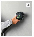
Once completely dry, sand the surface within the next day using a power or manual sander with a dry abrasive paper of P80 - P120 grit until the desired surface texture has been achieved.
