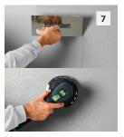
Note: depending on desired smoothness, additional coats of Stolit Milano and sanding may be required. Before each additional Stolit Milano application, blow/brush all lose particles from surface.
