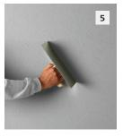
Apply a second thin layer of Stolit Milano in a similar manner as step 4 and smooth. Leave the surface to dry.
