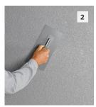
Float the freshly troweled finish in figure eight movements using a plastic float. Always remove any excess finish paste from the plastic trowel. Leave the surface to dry.
