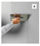
Using a stainless steel trowel, apply a thin coat of Stolit® Milano as a second layer to the dry Stolit 1.0. Only apply finish to the area that will be textured immediately.
