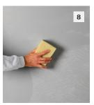
Wash the finished facade with clean water or carefully dust off dry.
