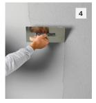
Using the stainless steel trowel, apply a thin layer of Stolit Milano to the dry Stolit 1.0. Let the finish dry. Knock the tips off the dried finish using the edge of the stainless steel trowel or lightly sand with P80 - P100 grit sand paper. Blow/brush all loose particles from surface.
