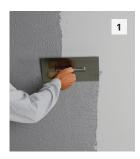
Using a stainless steel trowel, apply Stolit 1.0 and trowel off to aggregate size. Only apply finish to the area that will be textured immediately.
