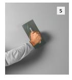
To create the texture, hold the trowel at a steeper angle. Trowel in a crisscross pattern to produce a finely rippled texture. Leave the surface to dry.
