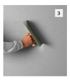
Knock the tips off the dried finish using the edge of the stainless steel trowel. Blow/brush all loose particles from surface.
