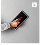
When the surface of the Stolit Milano starts to dry, float the entire surface with a slightly damp Sto-Rubber Sponge Float in a nondirectional manner. Leave the surface to dry.
