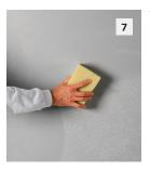
Wash the finished facade with clear water or carefully dust off dry. Optional: apply Sto Clear Coat Sealer of desired gloss.
