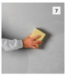
Wash the finished facade with clear water or carefully dust off dry. Optional: apply Sto Clear Coat Sealer of desired gloss.
