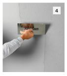
Using the stainless steel trowel, apply a thin, layer of Stolit Milano to the dry Stolit 1.0 with a steeper angle to produce a fine rippled texture. Let the finish start to dry.
