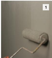
**1** Apply StoPrime UV over the basecoat. The primer is designed to remain exposed to open weather and will ultimately appear as mortar joints in the finished design. Allow to dry.
