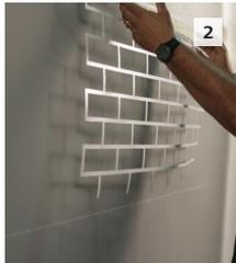
**2** Prior to placing the stencils, snap guidelines to ensure proper alignment, paying close attention to rough openings, corners and other details to achieve a final consistent appearance.
