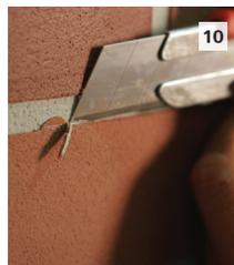
**10** If necessary, excess finish may be carefully removed with a flat scraper.
