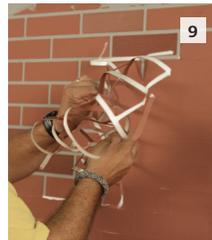
**9** Slowly remove each covered stencil, taking care to avoid damaging the finish that has been applied over it.
