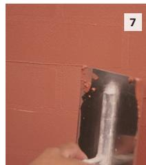
**7** Once the cells are completely filled, trowel the finish to the thickness of the aggregate size. Float the finish with a plastic trowel in a vertical motion to achieve the striated look.
