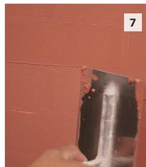
**7** Once the cells are completely filled, trowel horizontally along the mortar joints to ensure an even surface. Make sure to align the trowel on the mortar joint.
