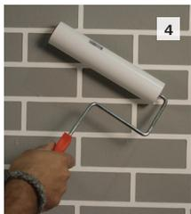
**4** Pass over the stencils with a paint roller and a PVC sleeve to help smooth out the stencil. Take caution if using a trowel as it may damage the stencil.
