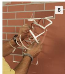
**8** When finish is completely dry, carefully remove the stencil to avoid damaging the finish.
