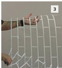
**3** Once the wall surface is properly laid out, remove the adhesive tape from the stencils and apply them to the surface in their designated positions.
