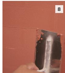
**8** Apply a second coat of the finish with a hopper sprayer or suitable spray equipment. Optionally, the second coat of finish may be applied with a trowel, then stippled using a trowel or textured roller. Once the finish is partially dry, smooth the finish in a horizontal or vertical manner with a knockdown trowel to achieve desired texture. Allow the finish to dry.
