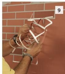
**9** When the finish is completely dry, carefully remove the stencil to avoid damaging the finish.
