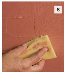
**8** Optional: when the finish is partially dry, a damp soft sponge can be used to create a fine finish.
