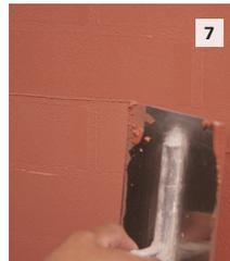
**7** Once the cells are completely filled, trowel horizontally along the mortar joints to ensure an even surface. Make sure to align the trowel on the mortar joint. Allow the finish to dry.
