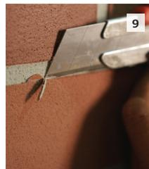
**9** If necessary, excess finish may be carefully removed with a flat scraper.
