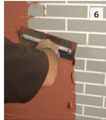
**6** When applying Sto Finish trowel in all four directions to ensure the stencil cells are properly filled.
