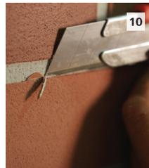
**10** Use a flat scrap to remove any excess finish from unclean edges.
