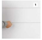
Install StoCast Brick units from top to bottom in accordance with the planned layout and start from a corner. Establish layout lines for the pattern in use.
