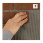
Press and gently slide the StoCast Brick units into the freshly applied mortar.
