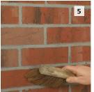
Once the adhesive has dried, clean the surface of the units using a suitable hand brush if necessary.
