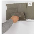
Starting from the top corner, apply Sto Bonding & Pointing Mortar using a  $\frac{1}{4} \times \frac{1}{4} \times \frac{1}{4}$  inch square notched stainless steel trowel and comb it vertically.
