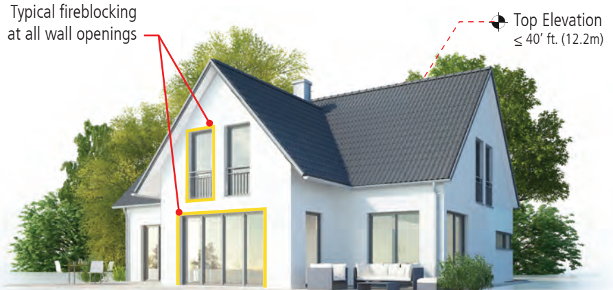
Figure 1.4 One-Family Detached Dwelling, Type V Construction.
