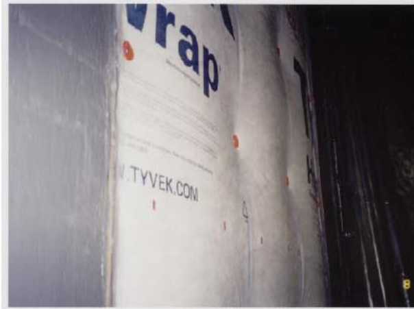
Figure 10. “Building Wrap A” specimen under negative wind loading conditions.
