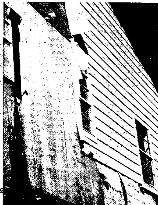
Figure 3 — Unfortunately, sill flashing is often omitted or incomplete beneath windows. The omission of flashing that would conduct window leakage to the exterior has caused wood rot beneath this window. Note that the presence of building paper and a housewrap material behind the siding failed to prevent water damage. The code must have clear, unambiguous requirements to prevent this problem. The window industry must play a role in developing such requirements.
