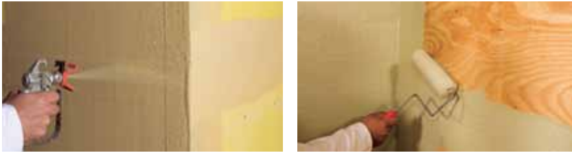
StoGuard can be applied with an airless sprayer or roller.
